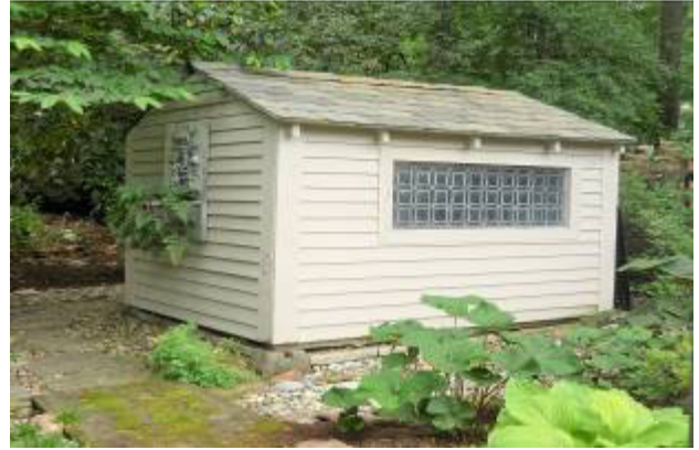
Beveled glass windows accent the side of what was once a chicken coop. Janelle now uses the structure as a tool shed.
